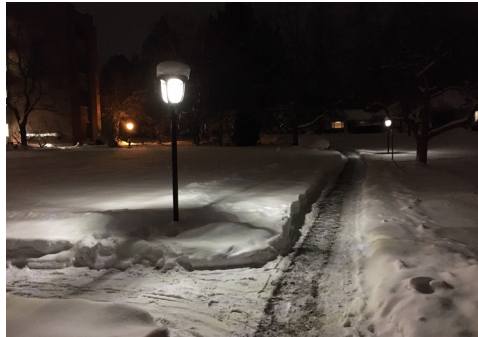
Sidewalk - 2000 Lumens Install Height = 6-7 FT
