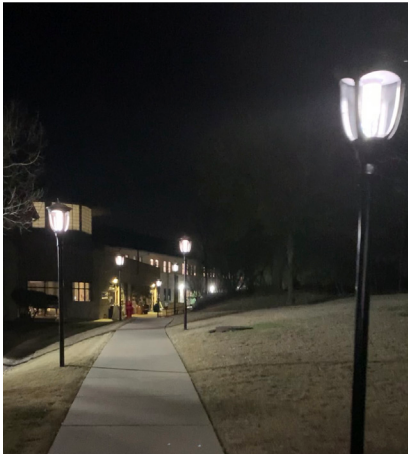
Sidewalk - 2000 Lumens Install Height = 6-7 FT
