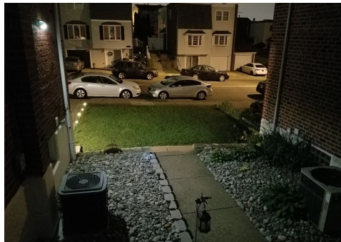
Pathway - 400 Lumens Install Height = 10 FT
