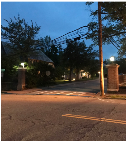
Street Pillars - 2000 Lumens Install Height = 6 FT
